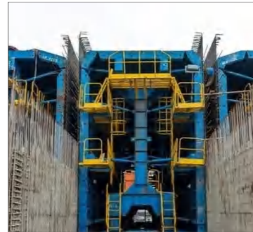
Steel Formwork Pipe Gallery Tunnel Trolley 钢模体系管廊台车
