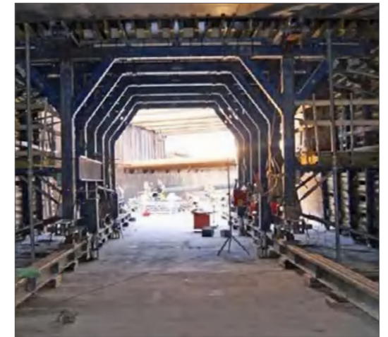
Timber Formwork Pipe Gallery Tunnel Trolley 木模体系台车
